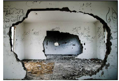
INTERIOR VIEW OF AN ABANDONED APARTMENT AFTER THE FIGHTING IN JENIN
