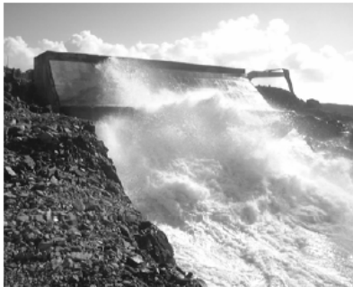
Figure 14-2 Shoreline OWC – the LIMPET Source: Wavegen
